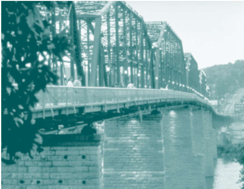
Restoration of this bridge in Chattanooga, TN helped to revitalize the city's under-used riverfront by allowing more pedestrian and bike use along the river.
