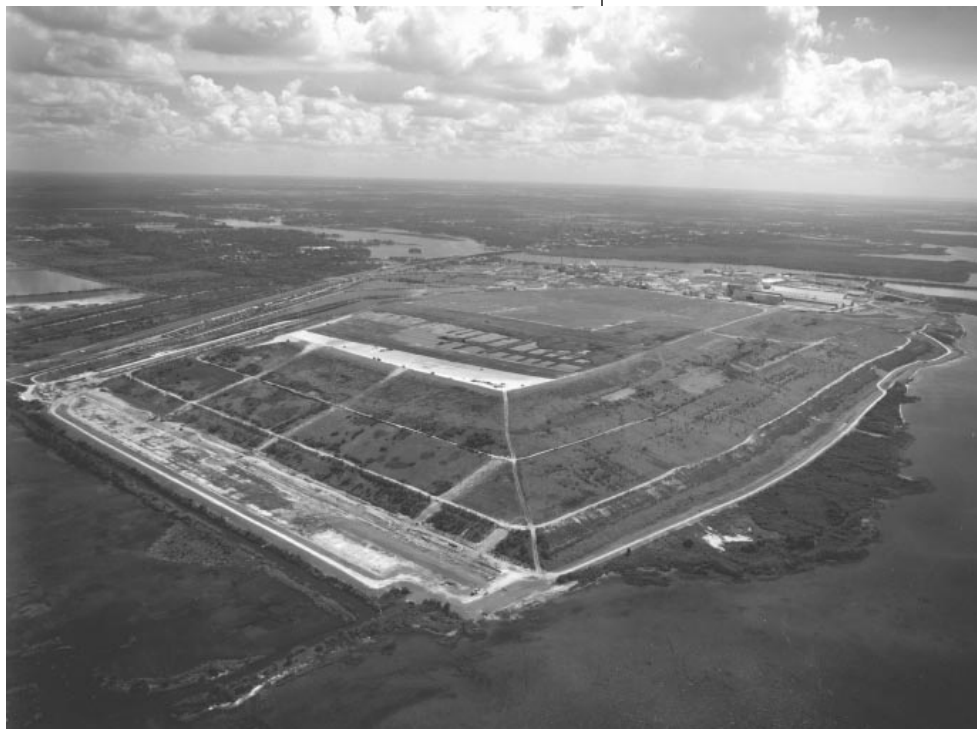
Closed phosphogypsum stack
